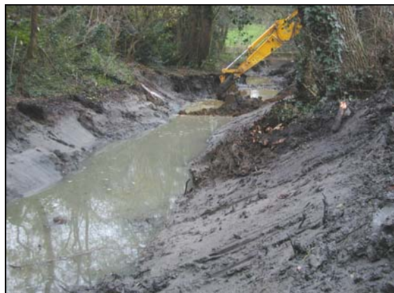
Plate VIII: desilting the moat
