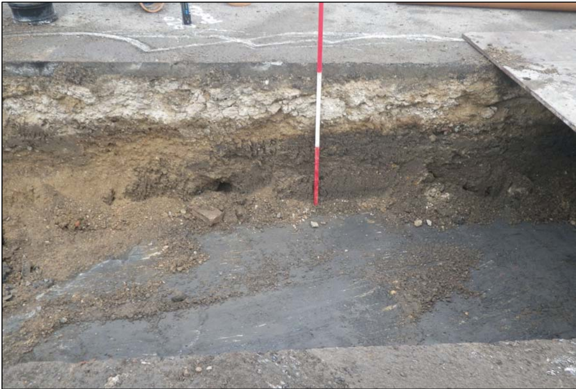
Plate 1. Concrete floor at west end of the building, camera facing north-east (ref. HSS 03)
