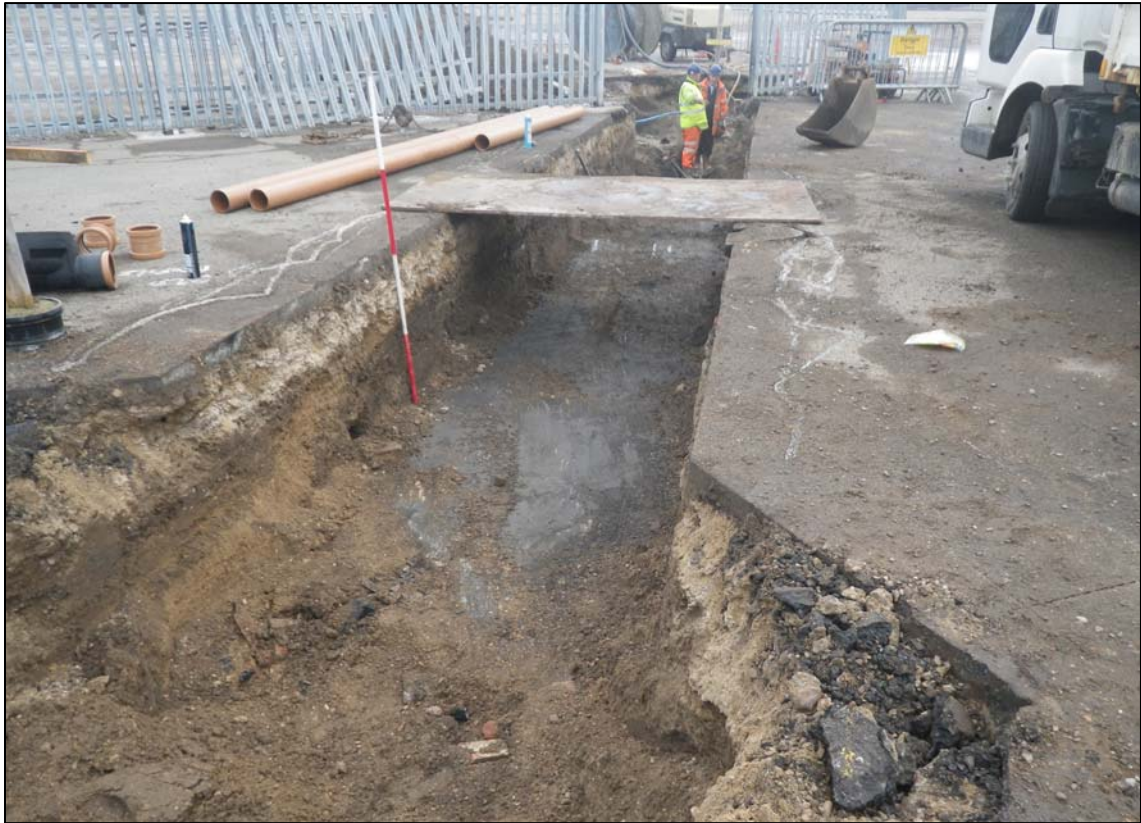
Plate 3. West end of the building, camera facing south east (ref. HSS 04)
